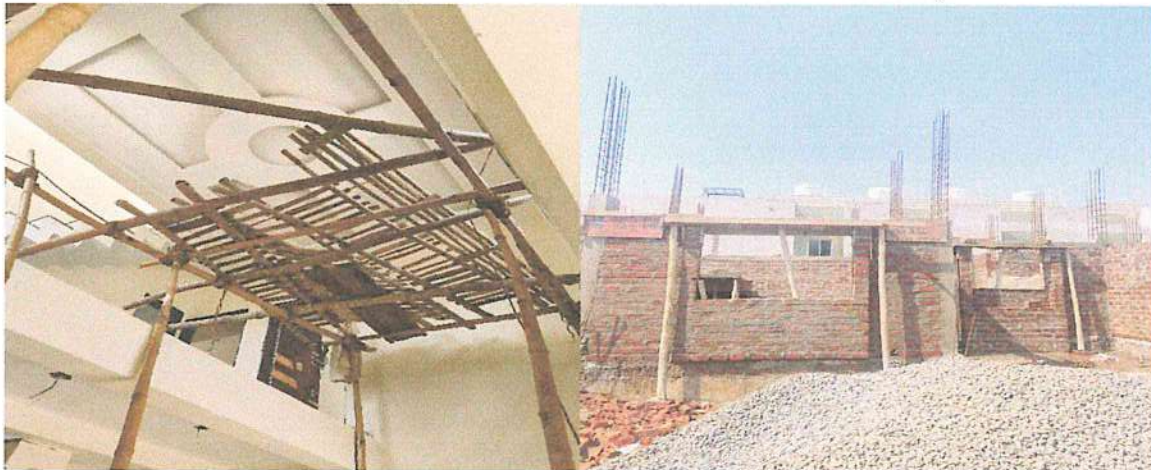
Fig. No. 5 Execution of Interior & Exterior of Construction Work
