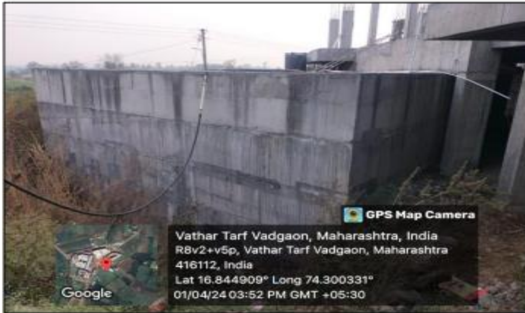
Fig 1: Water Storage Tank
